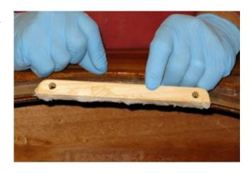
4. In they go, one block on either side of the hatch. These are about one inch from the bottom of the side panel.
